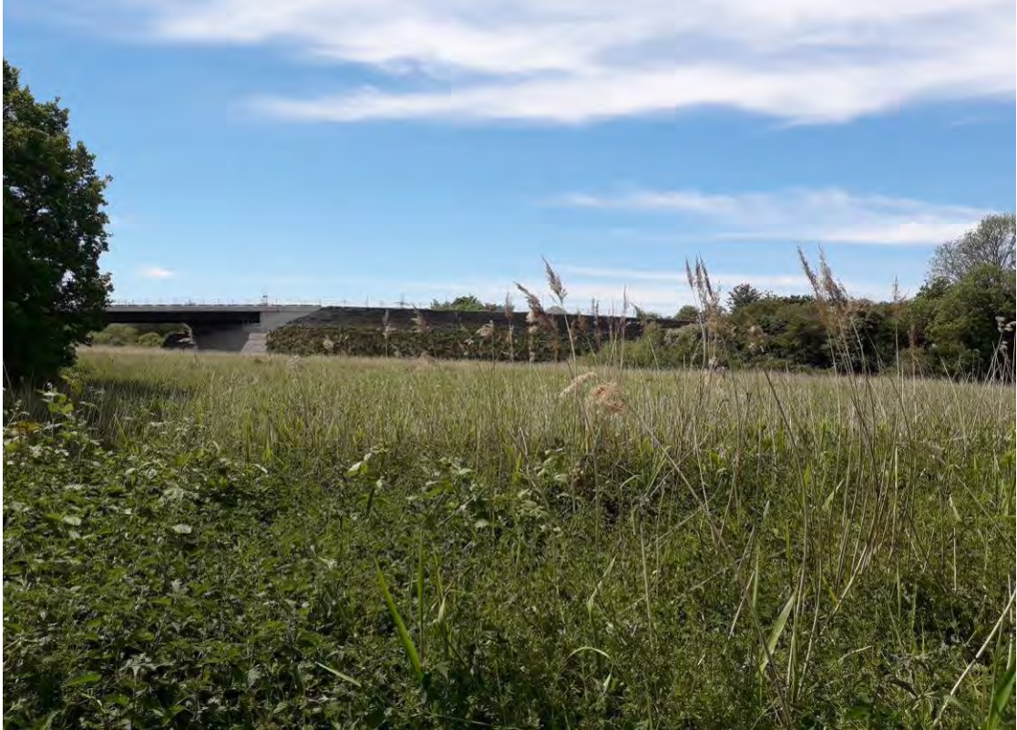
Image EDP A2.3: Section 2 - New construction spanning across River Ebbsfleet and associated wetland habitat.
