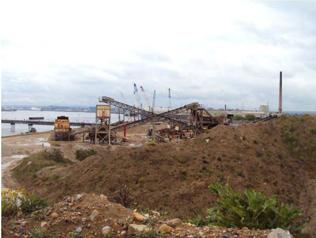
Figure A11 An area of active workings at TN21 with extensive areas of bare ground
